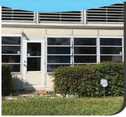
CURRENT TERRACE ENCLOSURE
